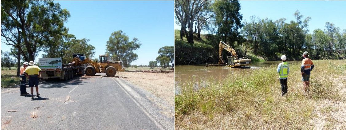
Plate 1 Logs being loaded onto the truck for transport to Macquarie River (left) and logs being placed in the river to create habitat for the nationally threatened Murry Cod (right)
